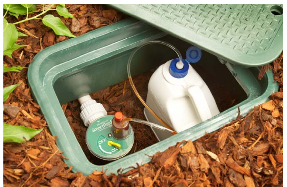
Figure 5: A properly installed SmartFeeder will look something like the illustration above. Notice that the valve box has been placed in the opposite direction of the irrigation system piping to make plenty of room for the fertilizer bottle. A jumbo valve box may also be used to accommodate larger fertilizer bottles for larger landscapes.
